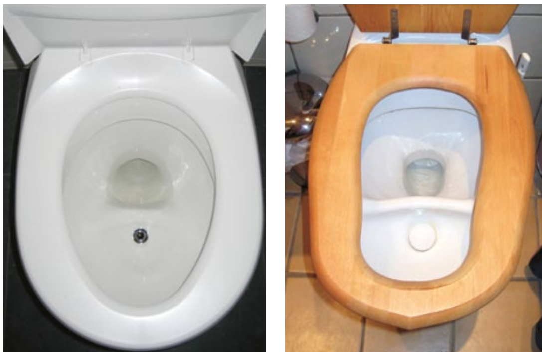
Figure 4.3.4.1 Urine diverting flush toilets. The left hand illustration shows an example from Meppel, the Netherlands; while the right hand illustration shows an example from Stockholm, Sweden.
